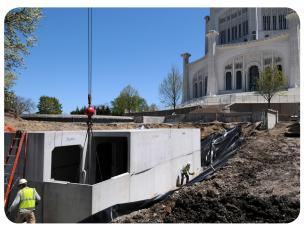
Baha'i Temple, Wilmette, Illinois Stormwater runoff flows into the 3048 mm StormTrap system and is harvested to irrigate the temple grounds. The DoubleTrap\* system holds over 141.584 m³ of rainwater.
